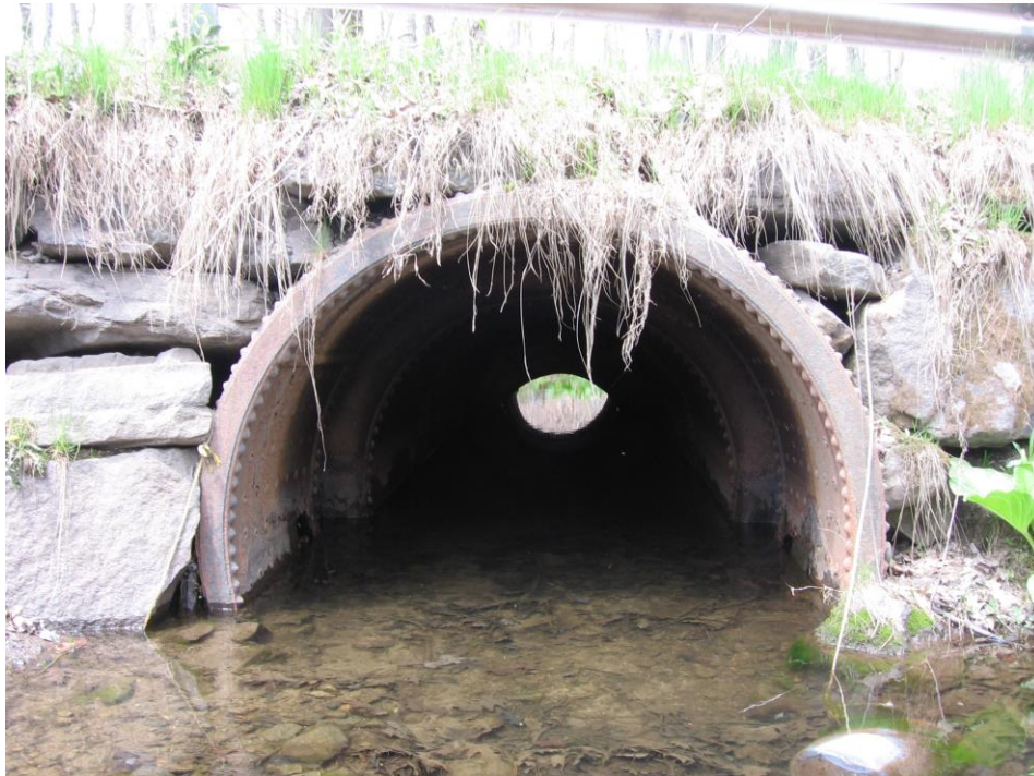
Note Pipe Size Change Under Roadway
