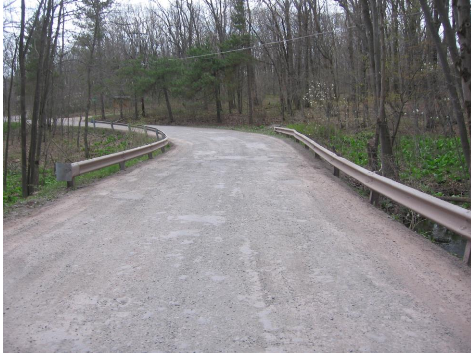
Existing Roadway over Culvert
