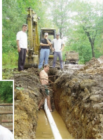
Photos courtesy of John Menichello. In the trenches, installing the dry hydrant.
